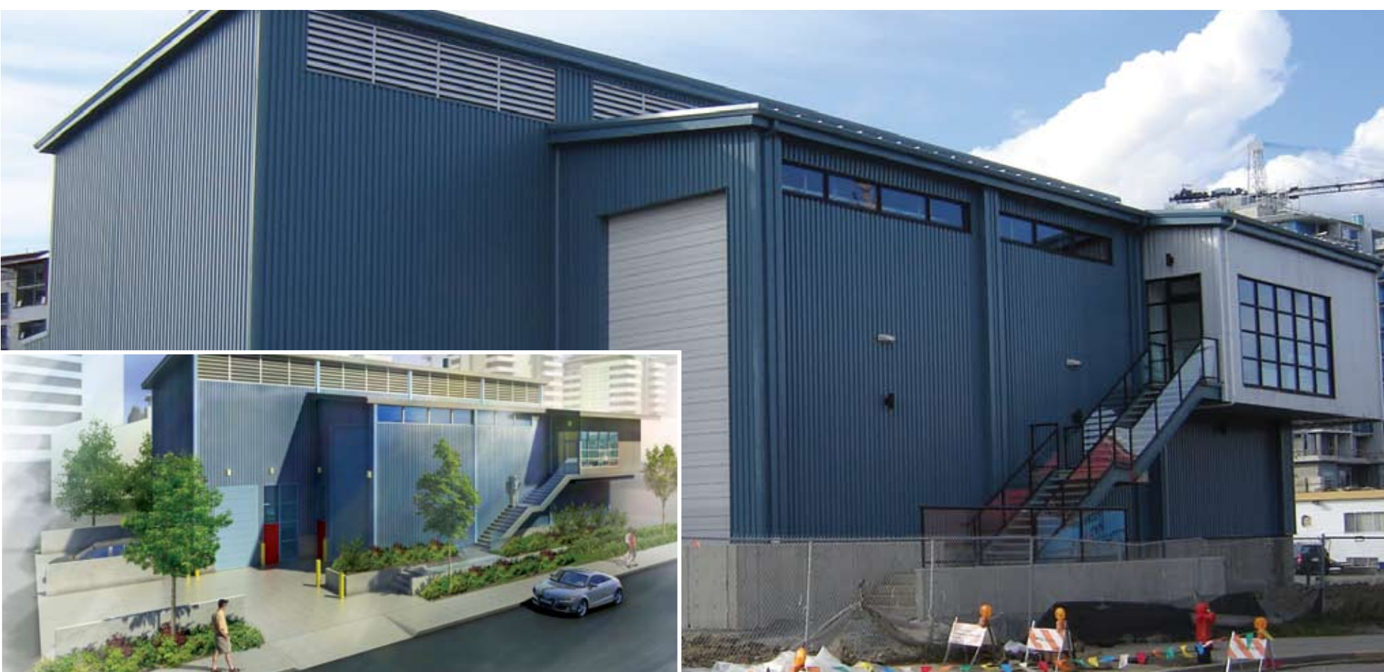
Dockside Green is a unique, sustainable community currently under development in Victoria and is North America's first community to target a Leadership in Energy and Environmental Design (LEED) Platinum status. The district energy system will be fuelled by locally-sourced wood waste to provide hydronic (water) energy to heat homes and domestic hot water.
